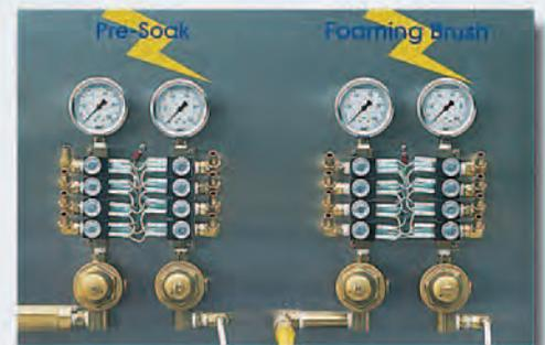
The low pressure control center is built with reliable pumps that include safety check valves, air and product regulators along with liquid filled pressure gauges.
